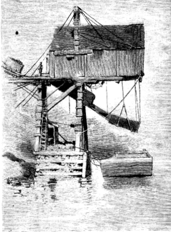
FIRST LOADING OF THE BARGE.
