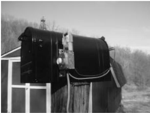
I lined the sides and back of the mailbox with 2 layers of frax insulation, and put one layer on the door. The door insulation is held in place with a scrap of metal grid and wire loops through the door.
