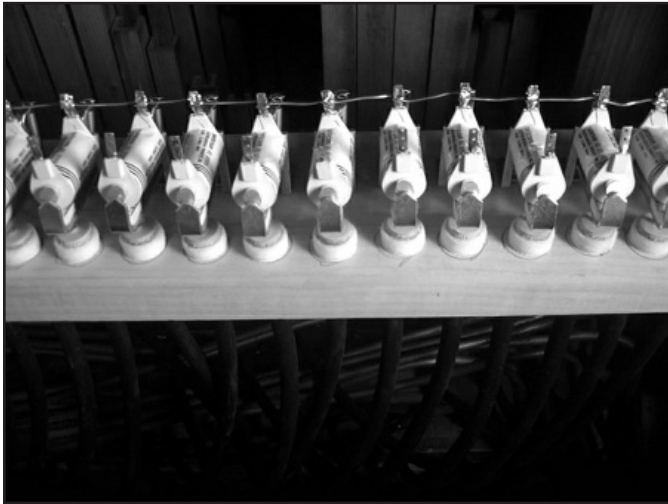
Figure 2. Manifold board from above showing the Peterson valves and the copper ground wire connecting each one together.
